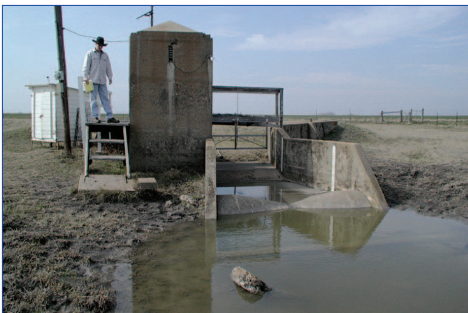
Figure 3. Field equipment to collect surface runoff.
